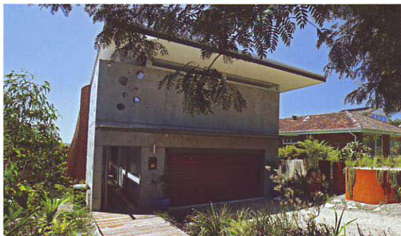
Burns/Soghomonian House Misho + Associates
